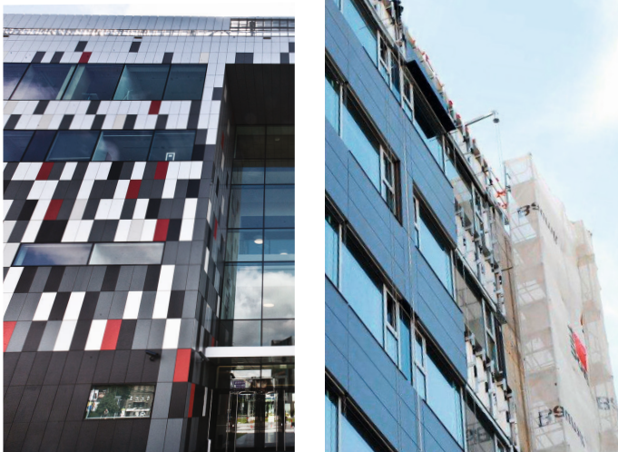
ICE Kraków Congress Center | Kraków, Poland Image courtesy of G Ziemianski
