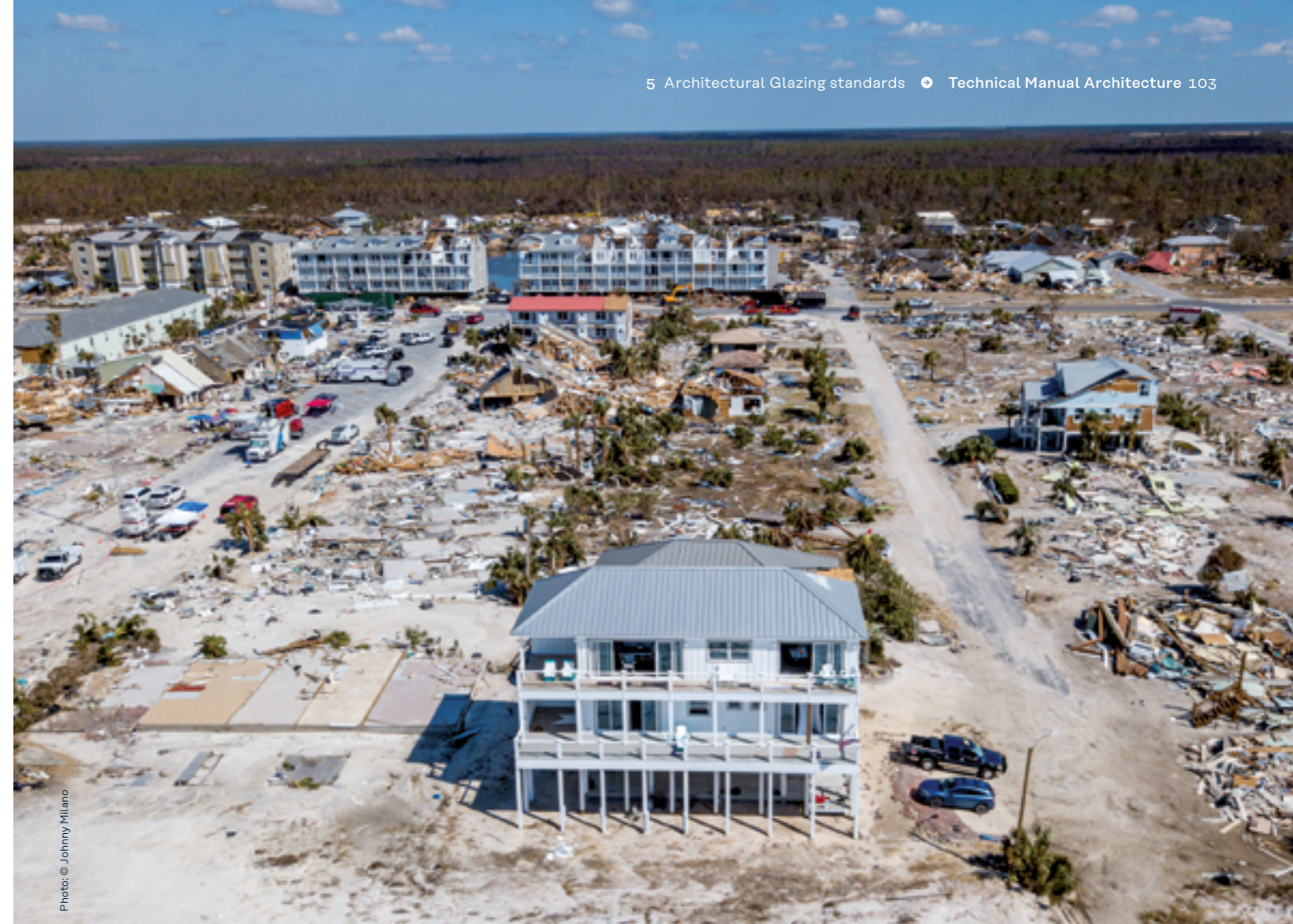
House still standing after Hurricane Michael 2018, Mexico Beach, Florida
