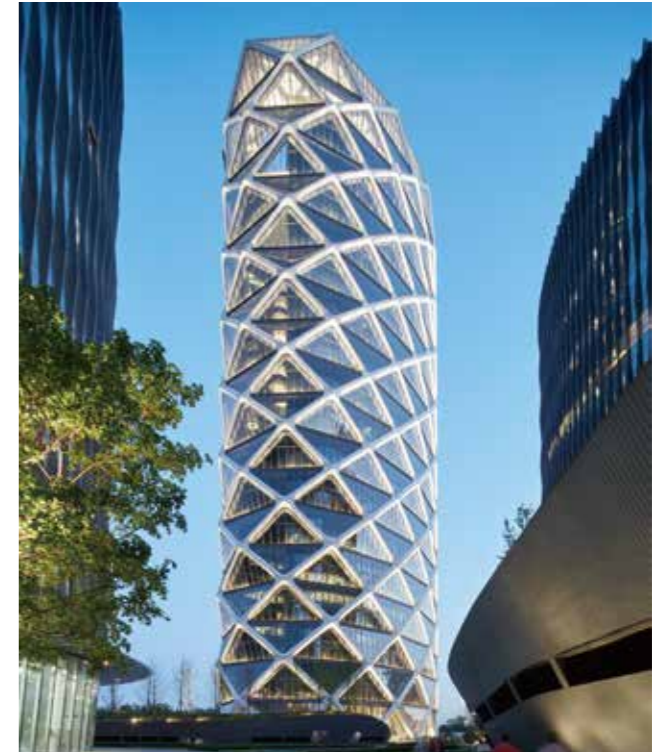
Beijing Baoli International Building
