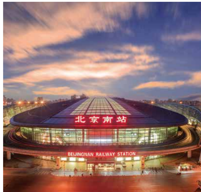
Beijing South Railway Station
