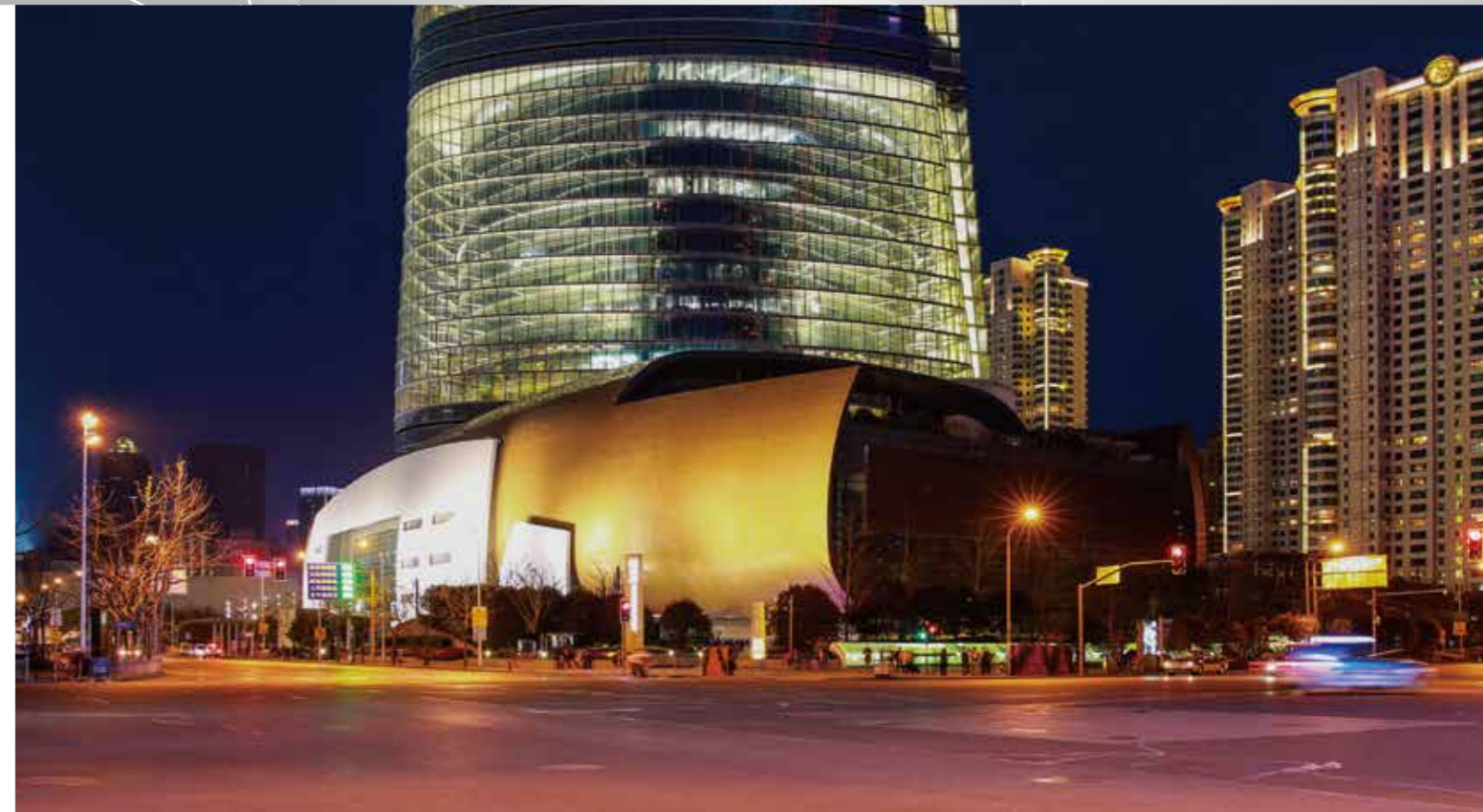
▲ Shanghai Tower Glass makeup: 6mm glazed glass HS +1.52 PVB + 6mm solar control coated glass (4#) +16mm AR + 6mm Clear glass + 0.38 PVB + 6mm clear glass Furnace used: B22S2536 & B15B8050
