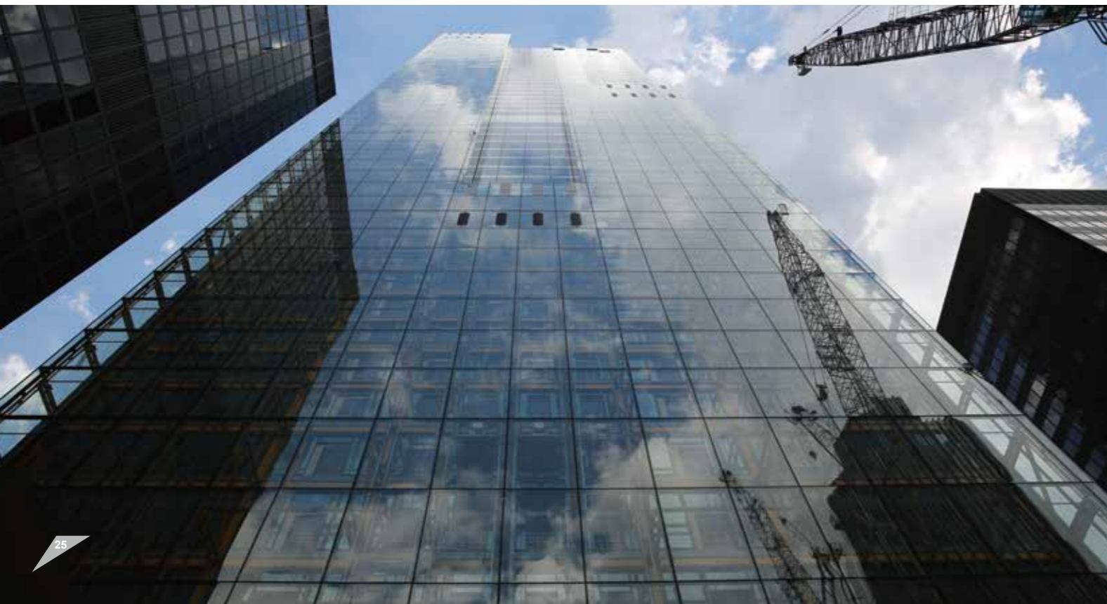
▼ London Leiden Building, UK Glass makeup: 6mm glazed glass HS+1.52PVB+6mm SunGuard SN51/28 Low-E glass HS (4#) +16mm AR + 6mm clear glass+0.38 PVB + 6mm clear glass Furnace used: AD1B80-GD
