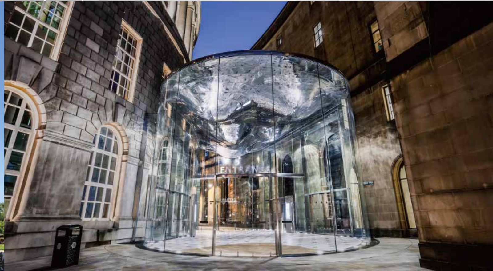
▲ Manchester Town Hall, UK Glass makeup: 3x12mm low iron glass curved tempered HST+2x1.52 SGP Furnace used: AC15E128
