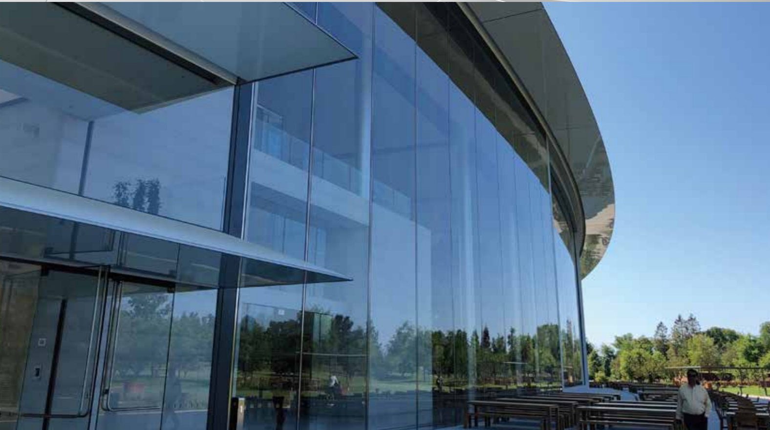
▲ Headquarters of the world's most famous consumer electronics company, US Furnace used: AU15M180, AG1T165
