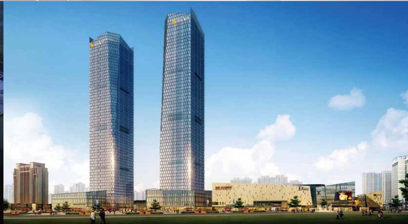
▲ Twin Towers in Xi'an Greenland Center Glass makeup: 10mm double-Ag Low-E coated glass+16mm AR+10mm clear flat glass tempered insulated+8mm double-Ag Low-E coated glass+16mm AR+8mm clear flat glass tempered insulated Furnace used: TG1B50
