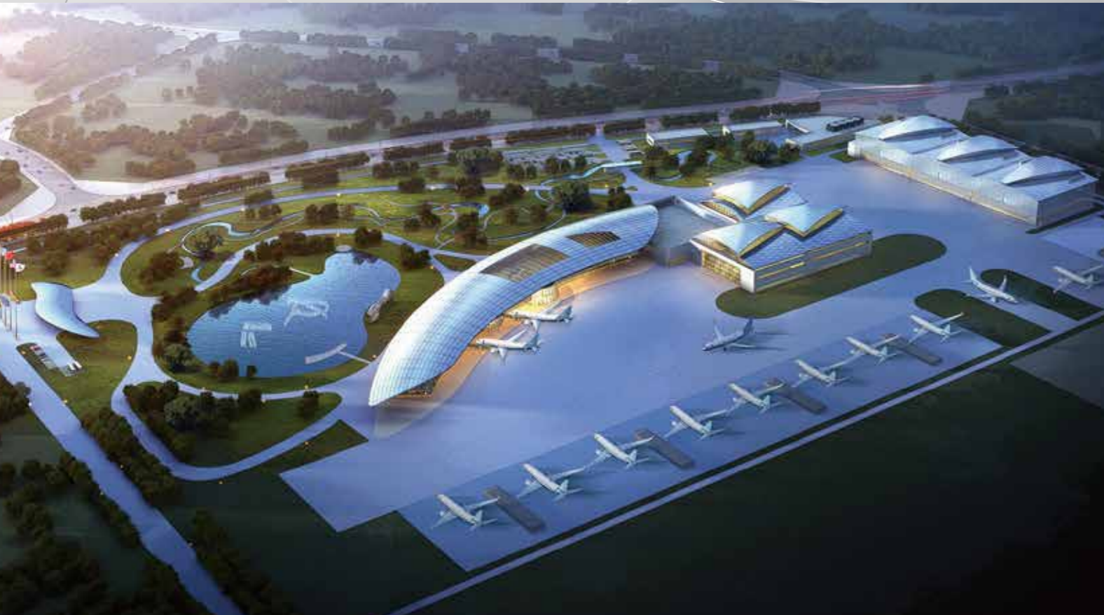
▲ Boeing 737 Delivery Center (Under Construction) Glass makeup: 10mm clear glass+2.28 PVB+10mm Low-E coated glass+16mm A+12mm dual curvature glass insulated Furnace used: AG22K2536 ( bending upwards & downwards )
